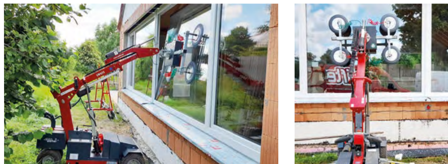
Suitable for outdoor use to move windows from the outside to the inside
